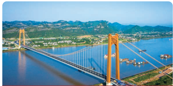
The Wujiagang Yangtze River Bridge in Yichang
