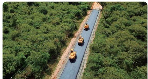
Upgrading and reconstruction of rural roads
