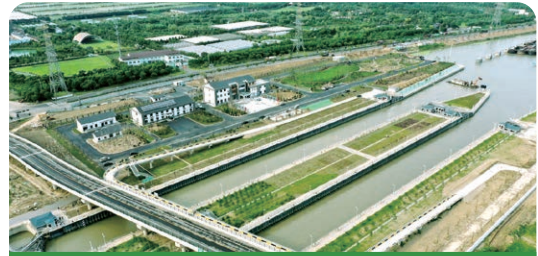
The Qianhuang junction of the Xinmeng River extension project
