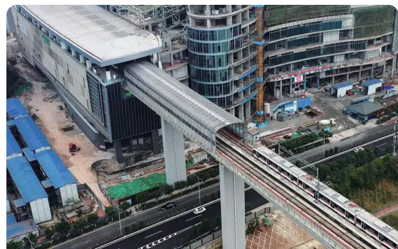
The first phase project of Chongqing Rail Transit Line 9
